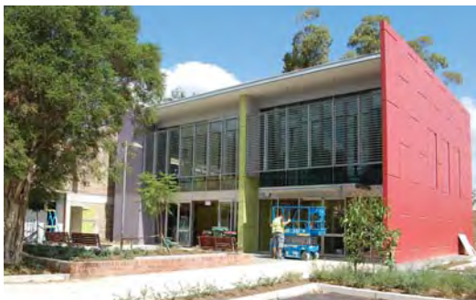
The new rear extension featuring two seminar rooms downstairs, and upstairs a students study area, local history room, periodicals reading lounge and balcony.
