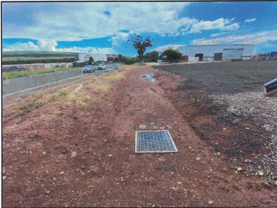
Photograph 4.0 – Grated Pit Outlet to the Detention Basin
