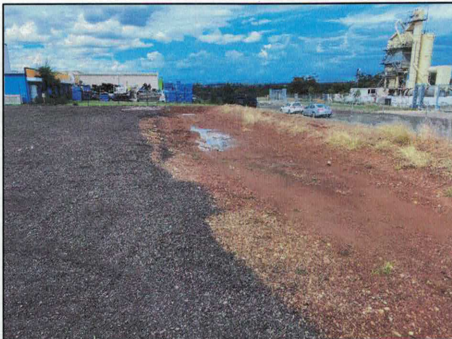
Photograph 3.0 – Constructed Detention Basin
