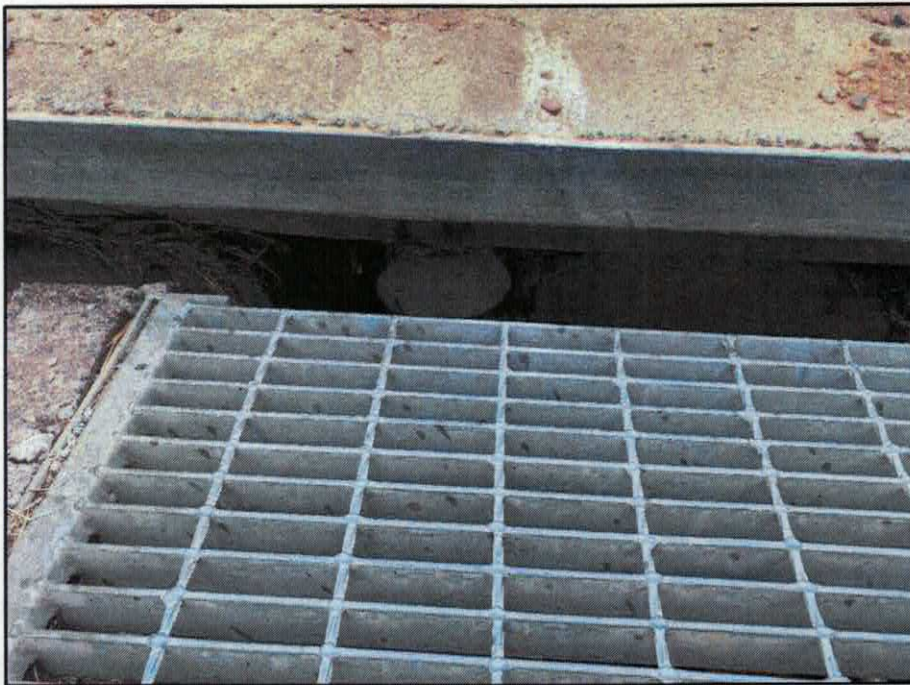
Photograph 5.0 – Site Outlet Pipe Connected into Existing Street Pit
