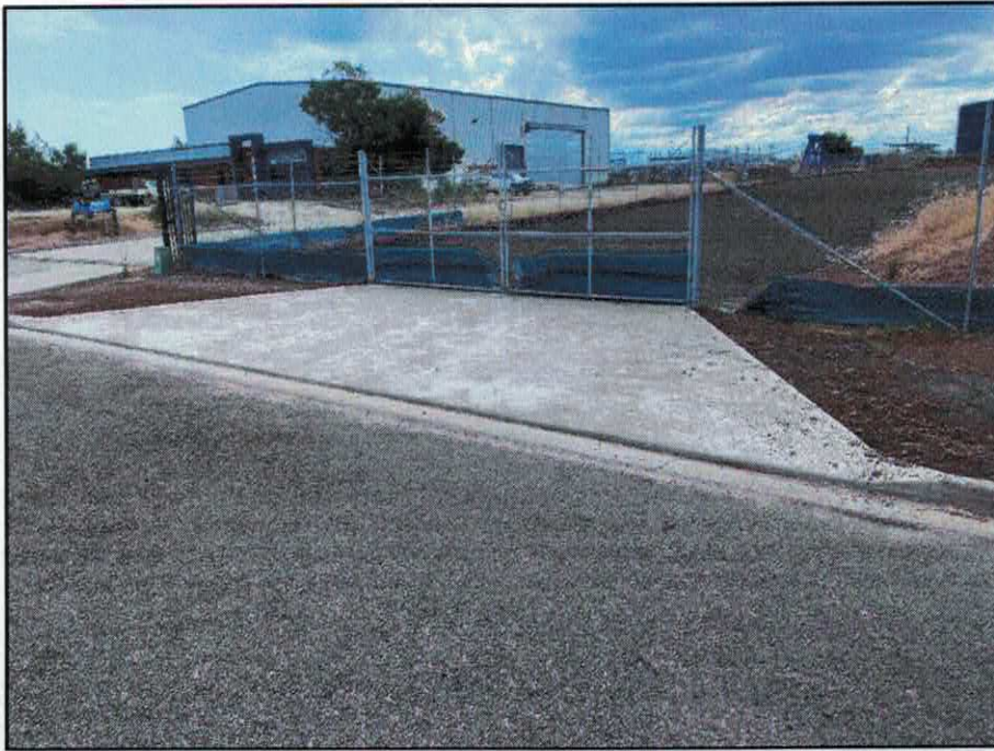
Photograph 2.0 – Access Driveway & Ramp off Enterprise Crescent
