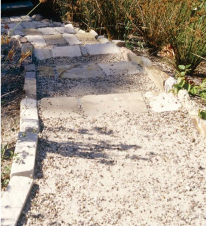
Stairs - sandstone and gravel with cement stabilisation
