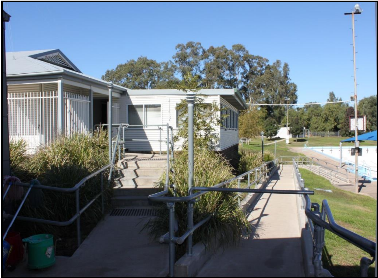
Figure 4: Existing office/amenities building - ramps and stairs to be removed with this building to be integrated within the proposed new pool hall
