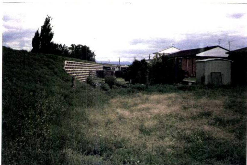
12. VIEW INSIDE THE LEVEE BANK SHOWING CRIBB WALL CONSTRUCTION Near Macauley Street.
