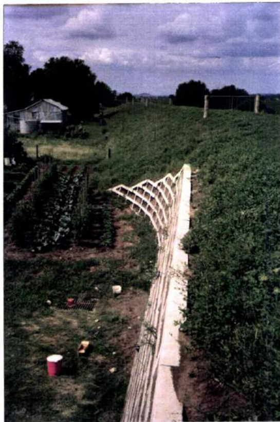
14. VIEW OF THE LEVEE BANK SHOWING 1:2 BATTER, CRIBB WALL AND INLET TO THE 375 mm dia CONCRETE DRAINAGE PIPE
