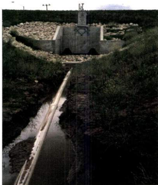
6. FLOOD CONTROL GATE WITH VERTICAL CONTROL GATE
