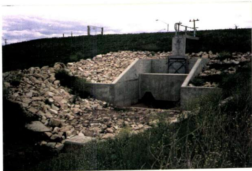
5. FLOOD CONTROL GATE WITH VERTICAL SLIDE GATE Near Crinoline Street.
