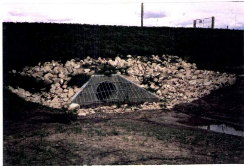
3. INLET TO FLOOD CONTROL GATE WITH TRASH RACK (1500 mm dia). Near Crinoline Street.
