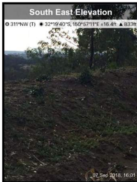
Photograph 4: The revegetated dirty water containment and diverting bank that is constructed along the western side of the quarry. It is approximately 1 metre high and has a batter of 2:1.
