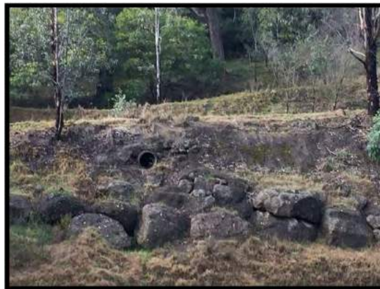
Photograph 13: Rock Flume Drop Structure Directing clean water runoff from the concrete culvert outlet under The Haulage Road to Sediment Dam 13.
