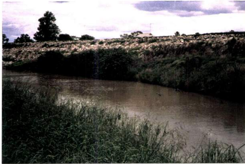
11. VIEW OUTSIDE THE LEVEE SHOWING BANK PROTECTION Sandy Creek in the foreground. Near Ogilvie Street.
