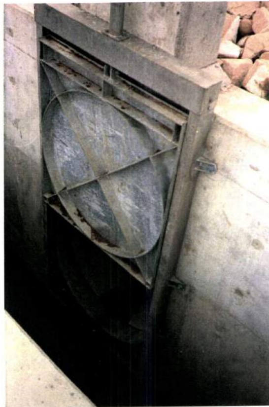
7. VIEW OF VERTICAL SLIDE GATE NEAR CRINOLINE STREET
