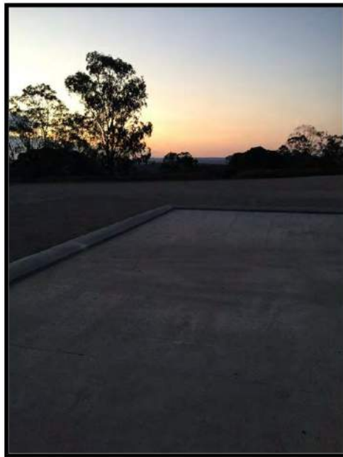
Photograph 24: Mobile Cement Batching Plant. Close up of the Concrete Walled Area to catch any spillage. This structure is also the top of the in-ground spillage containment tank that is regularly pumped out, so any spillage will be contained on site with in the tank.
