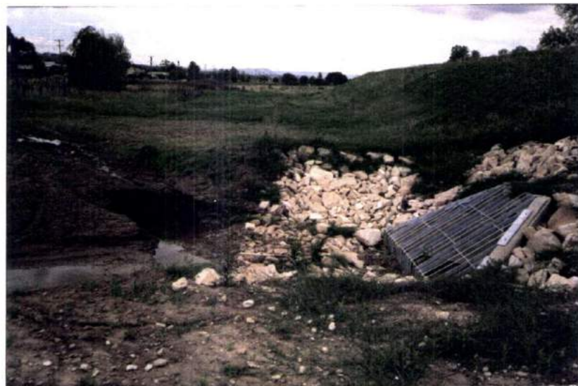
4. VIEW OF INLET TO FLOOD CONTROL GATE Near Crinoline Street. Note: Erosion due to drainage after heavy rain.
