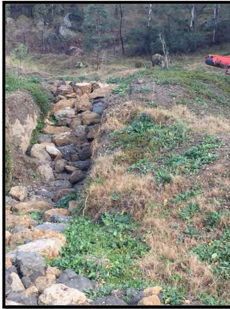
Photograph 12: Rock Flume Drop Structure directing clean water runoff to a concrete culvert under The Haulage Road.
