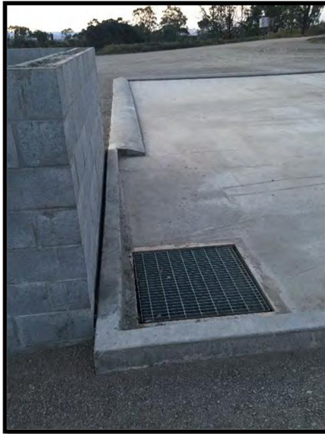
Photograph 25: This is the sump that directs spillage water from the concrete pad into the under-ground storage containment tank.
