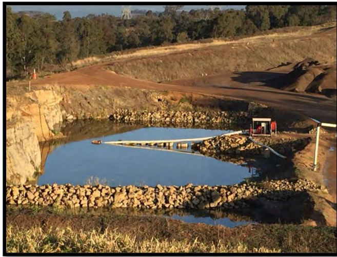
Photograph 1: Sediment Dam 1 in Quarry in Pit Area – Note sediment is pumped to Sediment Dam 2 if this dam is at capacity to ensure it has detention capacity.
