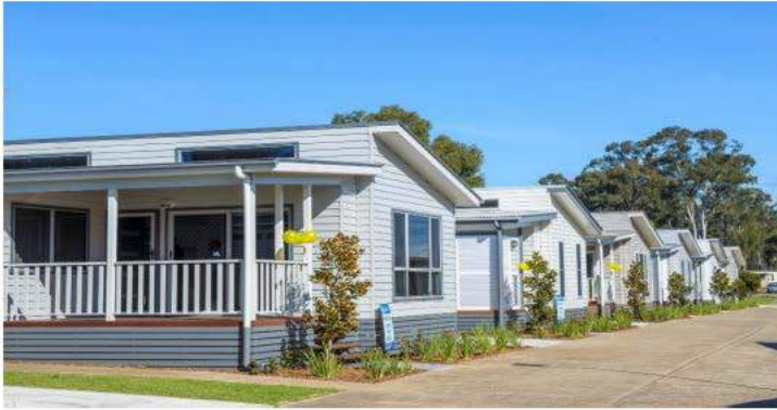
Figure 1.3: Photo showing a row of modular manufactured homes constructed offsite and transported in. Note: typical treatment of elevated floors requiring subfloor and stairs for access
