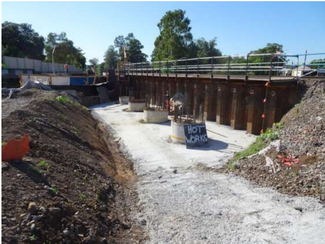
Pile Cap - North Western side of Bridge St – Note Temporary sheetpiles supporting track - January 2021
