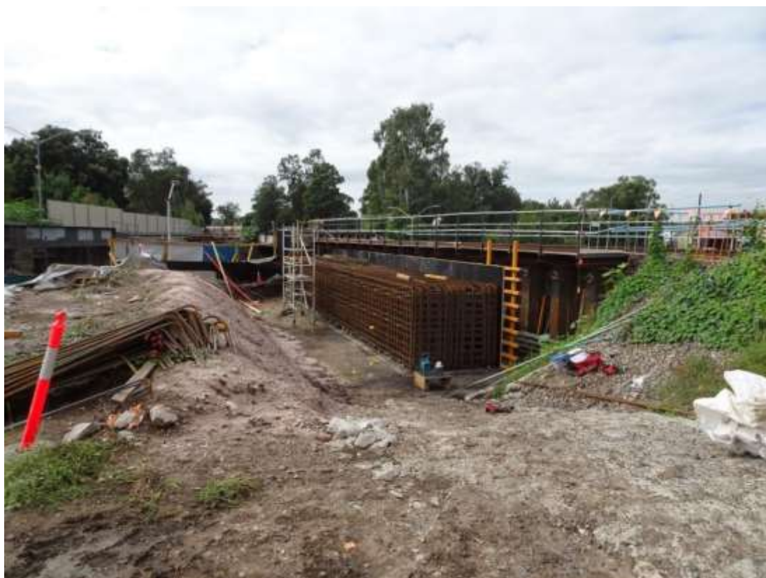
Pile Cap – North Western side of Bridge St – Steel Fixing – March 2021
