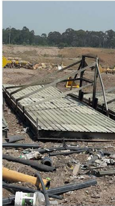
Figure 2: Lid 1. Exposed and burnt insulation, charring and displacement of sheeting. Lid no longer provides effective cover of waste.
