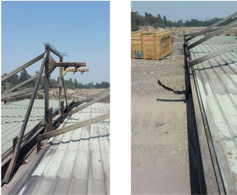
Figure 9: Lid 5 (left) lifting assembly, Lid 6 (right). Paint/galvanising either charred or burnt off.
