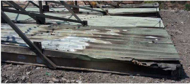
Figure 7: Lid 4 intense heat damage to sheeting & steel frame.
