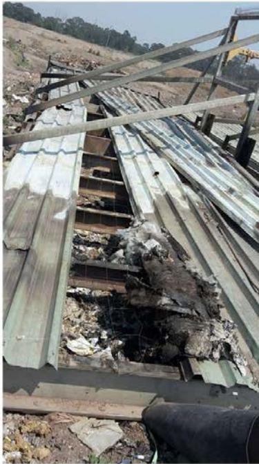
Figure 2: Lid 1. Exposed and burnt insulation, charring and displacement of sheeting. Lid no longer provides effective cover of waste.
