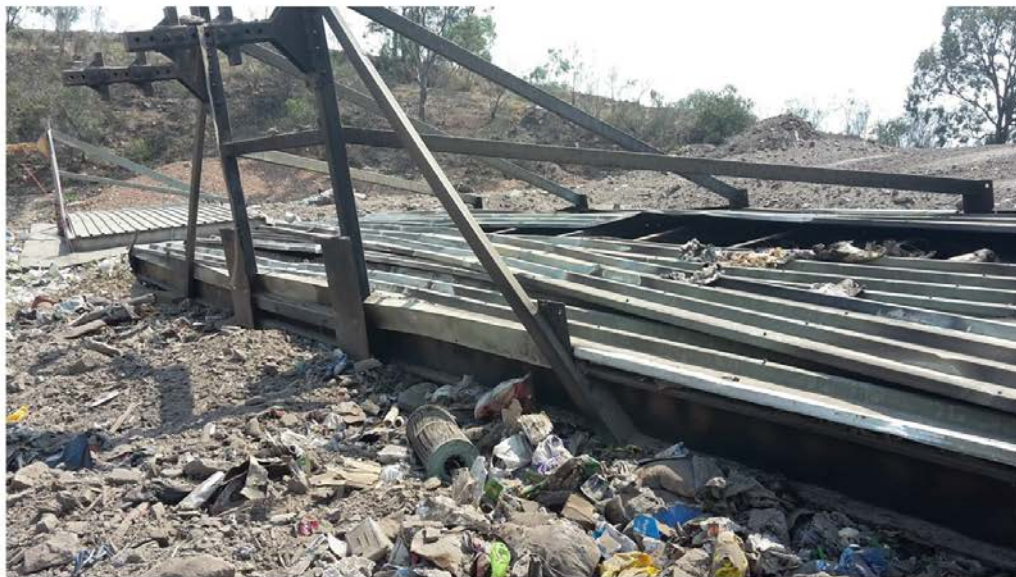
Figure 13: Lid 7 (foreground) and Lid 8 (background). Lid 7 appears in very poor condition with charring of steel lifting assembly evident. Lid 8 in the background was not in use on waste when the fire occurred and is in fair working condition with no notable damage and skirts intact.
