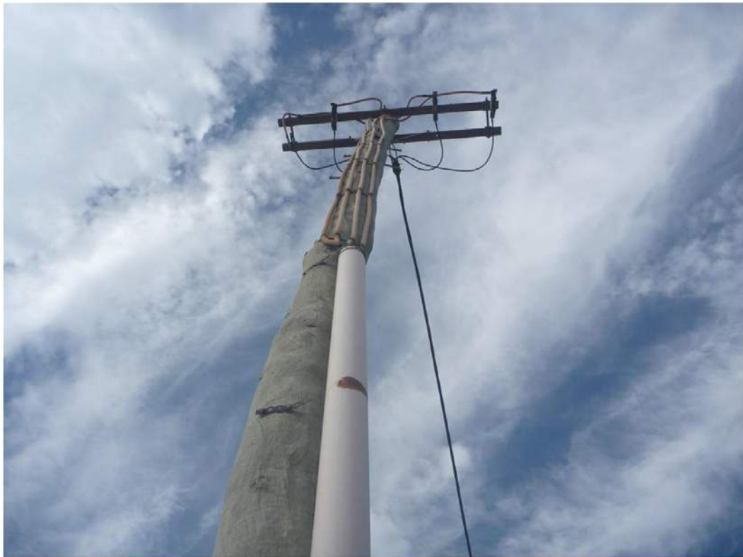
Figure 1 - Existing Service Pole that supplies the Site (Service Fuses can be seen atop the pole)
