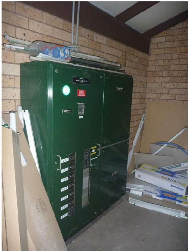
Figure 2 – Existing Main Switchboard (MSB)
