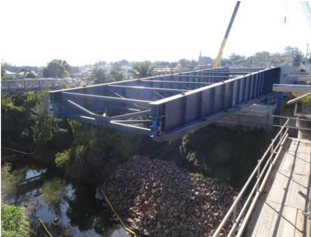
Superstructure segment 1 launched.
