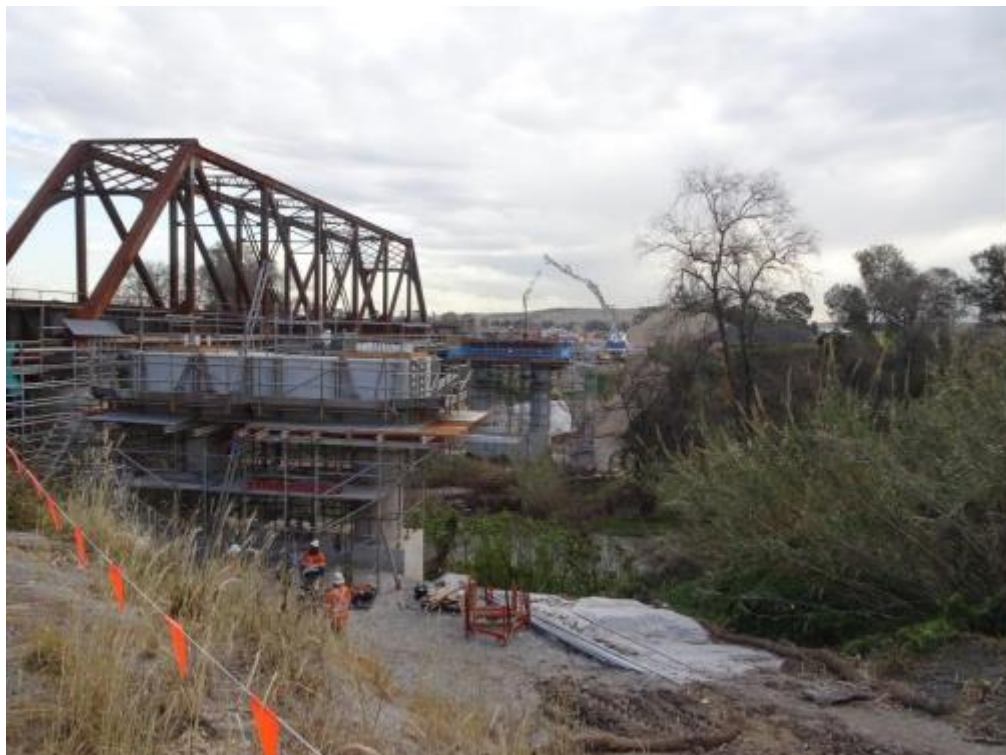
Pier 2 and Pier 3 of the new bridge. Pier 3 Headstock being poured in this picture. Hunter river flows between these two piers.
