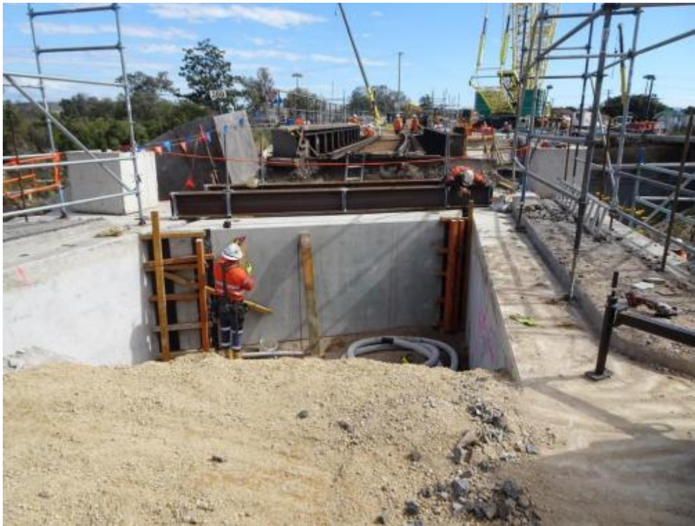
Abutment beam in position. Note – concrete beams on either side are the deflection wall pile caps.
