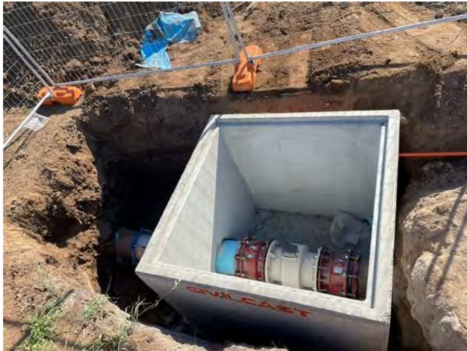
Figure 3 Denman Raw Water Main Flowmeter Installation
