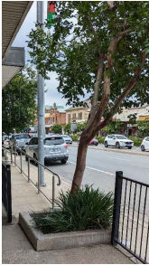
Planting pocket with concrete kerb
