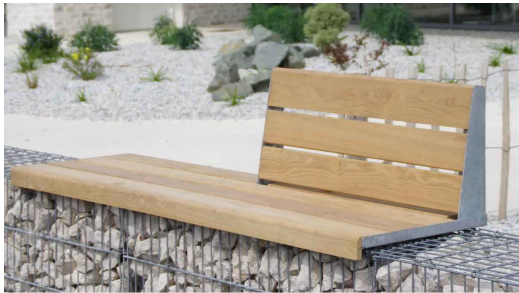
Pocket Park: Gabion seating wall with timber top
