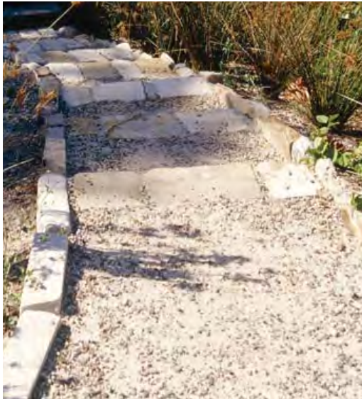
Stairs - sandstone and gravel with cement stabilisation
