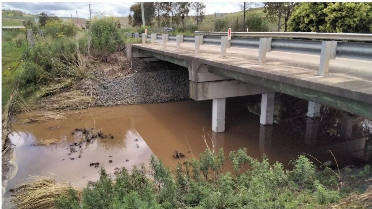
Plate 7. Rosebrook Bridge, view to west side of bridge, showing stabilisation works and cut into creek bank
