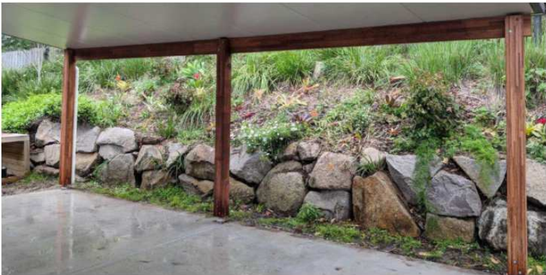
INSULATED PANEL ROOF WITH COLORBOND SOFFIT - HARDWOOD POSTS AND BEAMS
