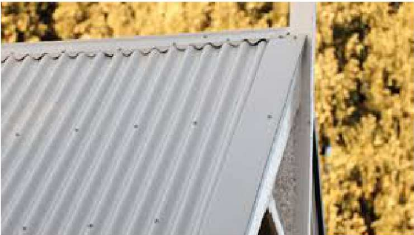
COLORBOND SHALE GREY ROOFING IN CUSTOM ORB
