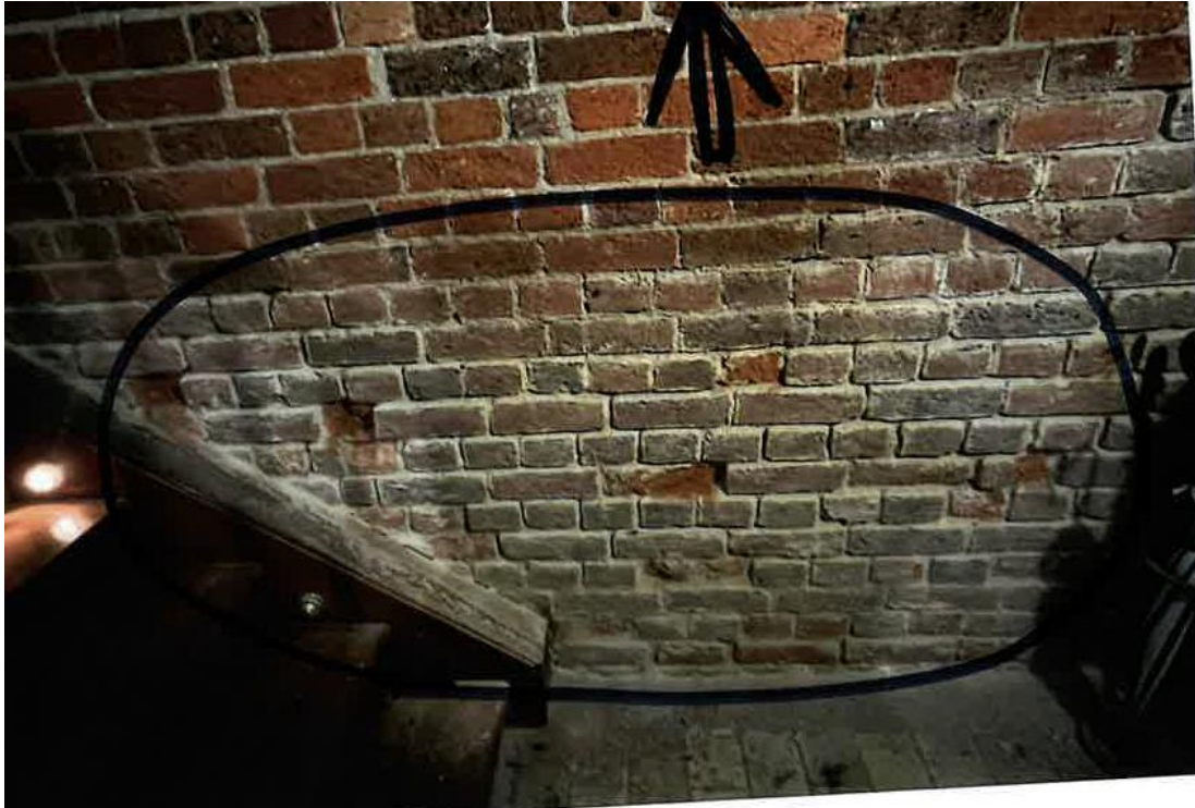
Image 2. Bricks and mortar requiring repair at 33 Brentwood Street, Muswellbrook.
