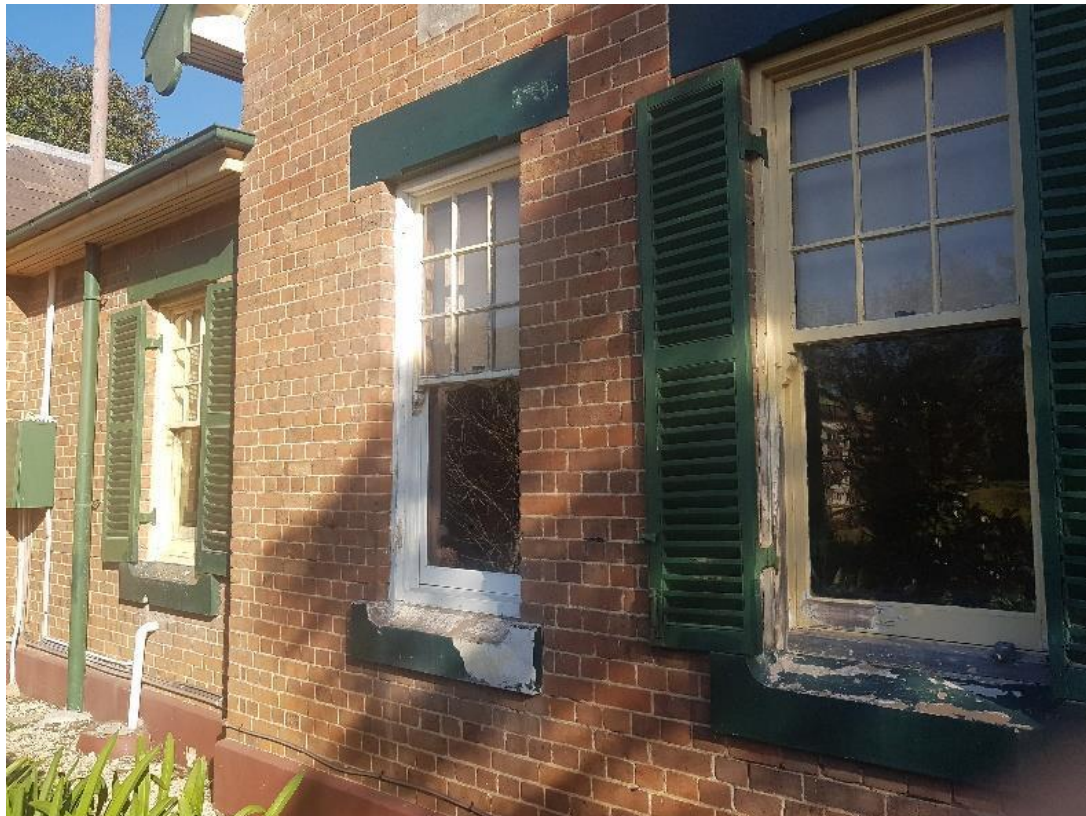
Image 1. Windows to be repaired 5 Midanga Ave, Muswellbrook
