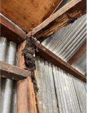
Structural timber framing in the unlined rear extension is damaged from termite attack
