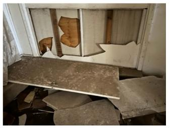
Internal fibro wall & ceiling lining throughout the shop, likely to be asbestos, is damaged in many locations.
