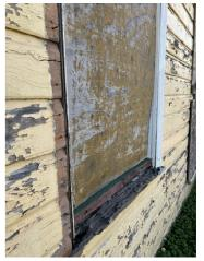
Timber framed windows are deteriorated throughout, including this rotten east side window sill.
