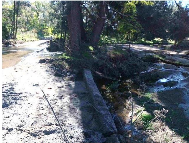
Photo 3: Washed away bench downstream of causeway
