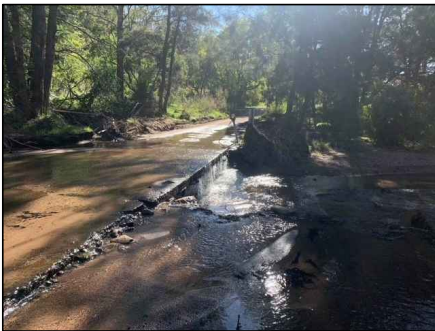
CAUSEWAY, SPILLWAY & DAMAGED APRON
