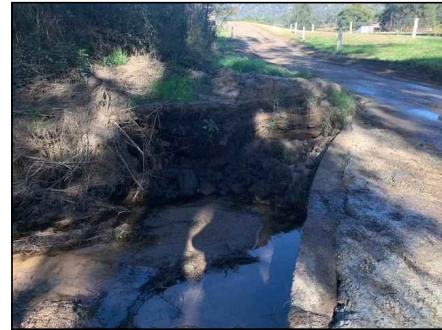
OUTFLANKING OF CAUSEWAY - IMMEDIATELY DOWNSTREAM - RIGHT BANK
