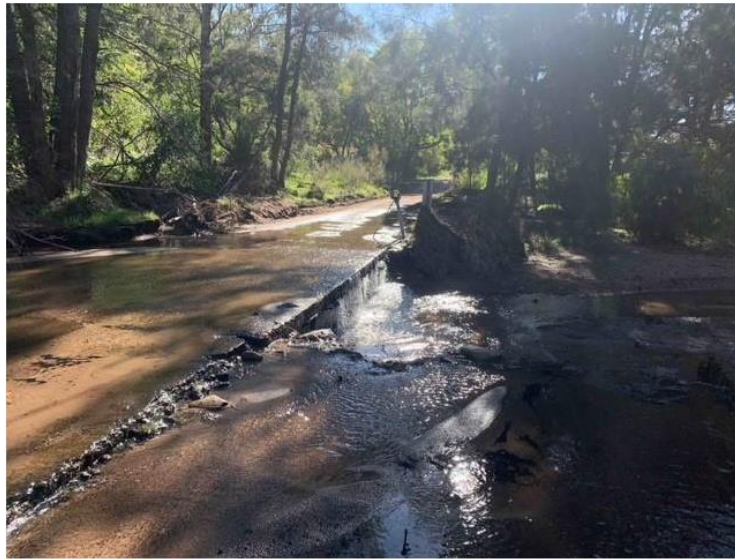
Photo 1: Damaged causeway and apron
