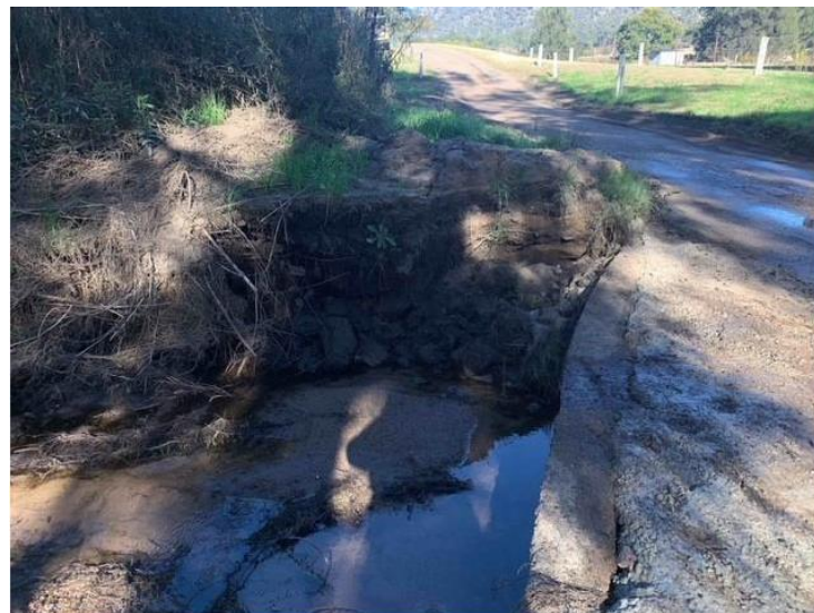
Photo 2: Outflanking of causeway right bank
