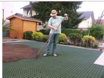
Figure 2-16: Grass pavers install (All Stake Supply, n.d.)
