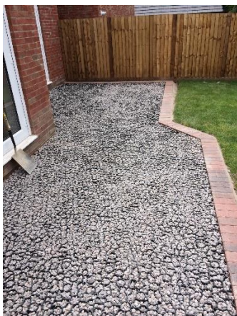
Figure 2-18: Gravel pavement residential installation (MatsGrids, 2015)
