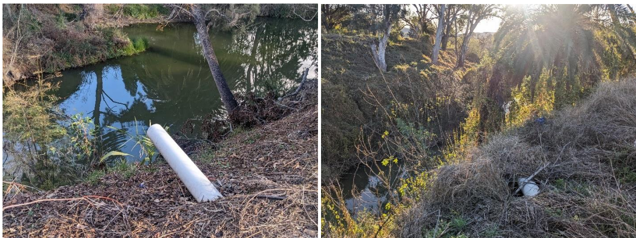
Figure 2-5: Stormwater outlets that do not have adequate scour protection, therefore causing bank scour. Examples given are located in reach 3 (left) and reach 4 (right).
