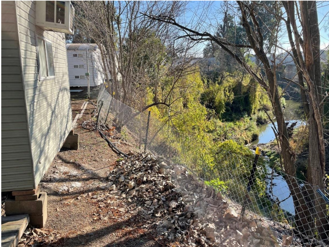
Figure 7-44: Caravans located immediately at the top of steep, high unstable creek bank.
