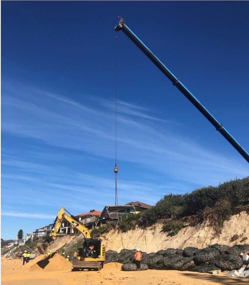
Figure 7-40: Rock bags being craned over properties during placement, Wamberal, NSW.
