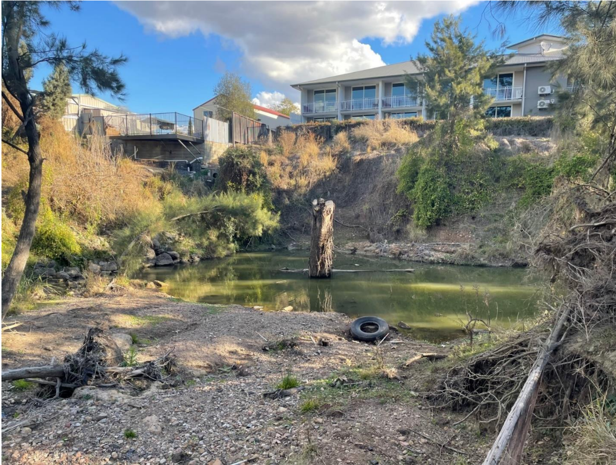
Figure 7-37: Creek bank erosion at Motor Inn site, looking downstream from right hand bank.
