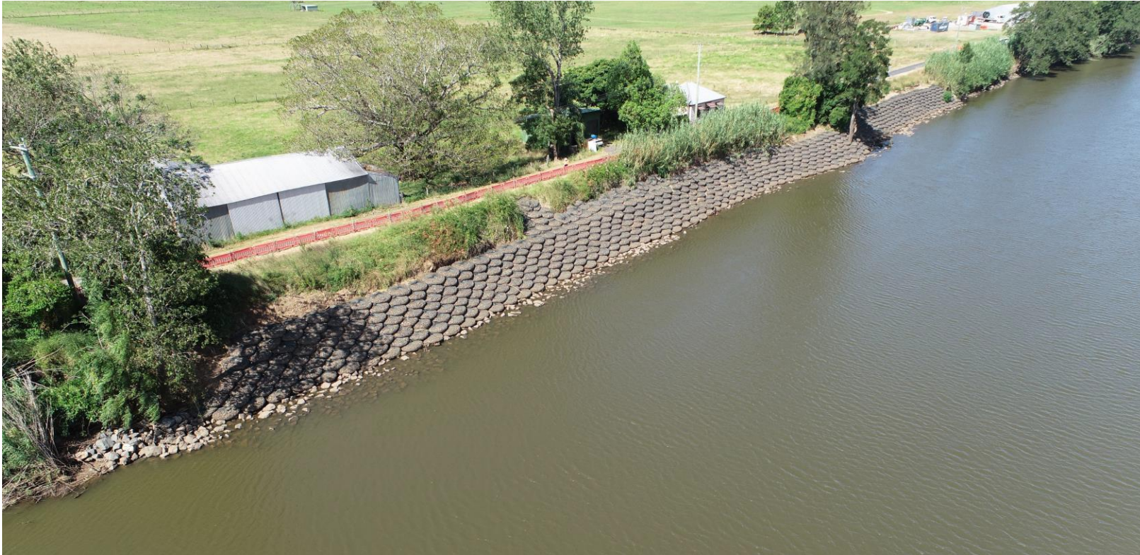
Figure 7-39: Rock bags used to provide short term riverbank stabilisation at Morpeth on the Hunter River.
