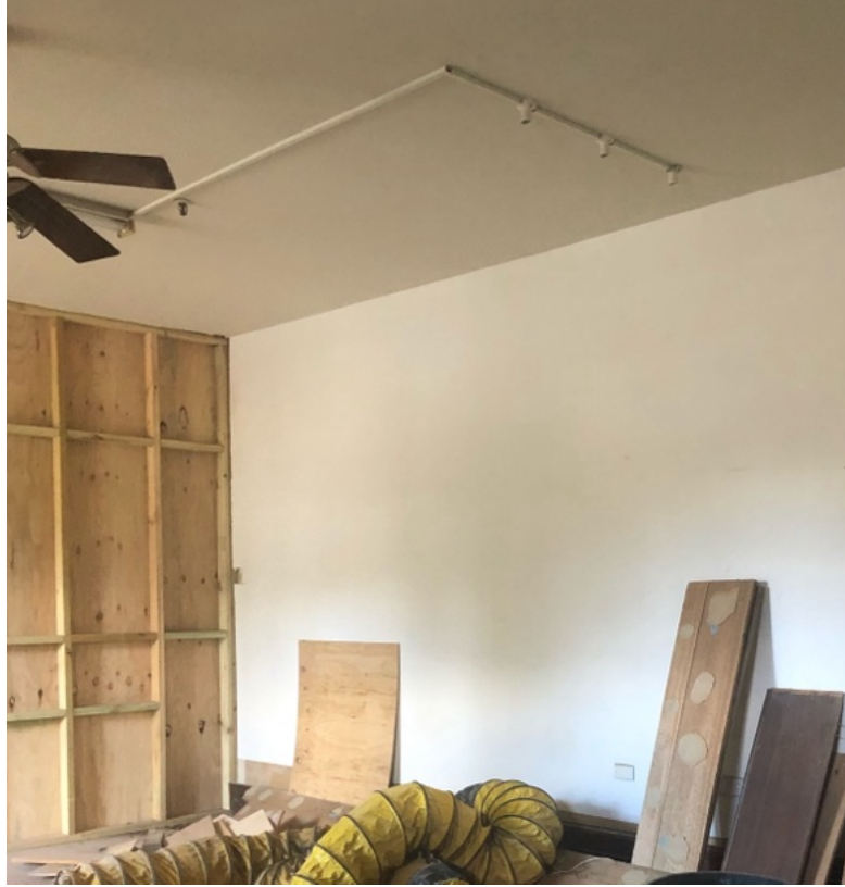
Evidence of plasterboard/stud partitions in ground floor rooms
