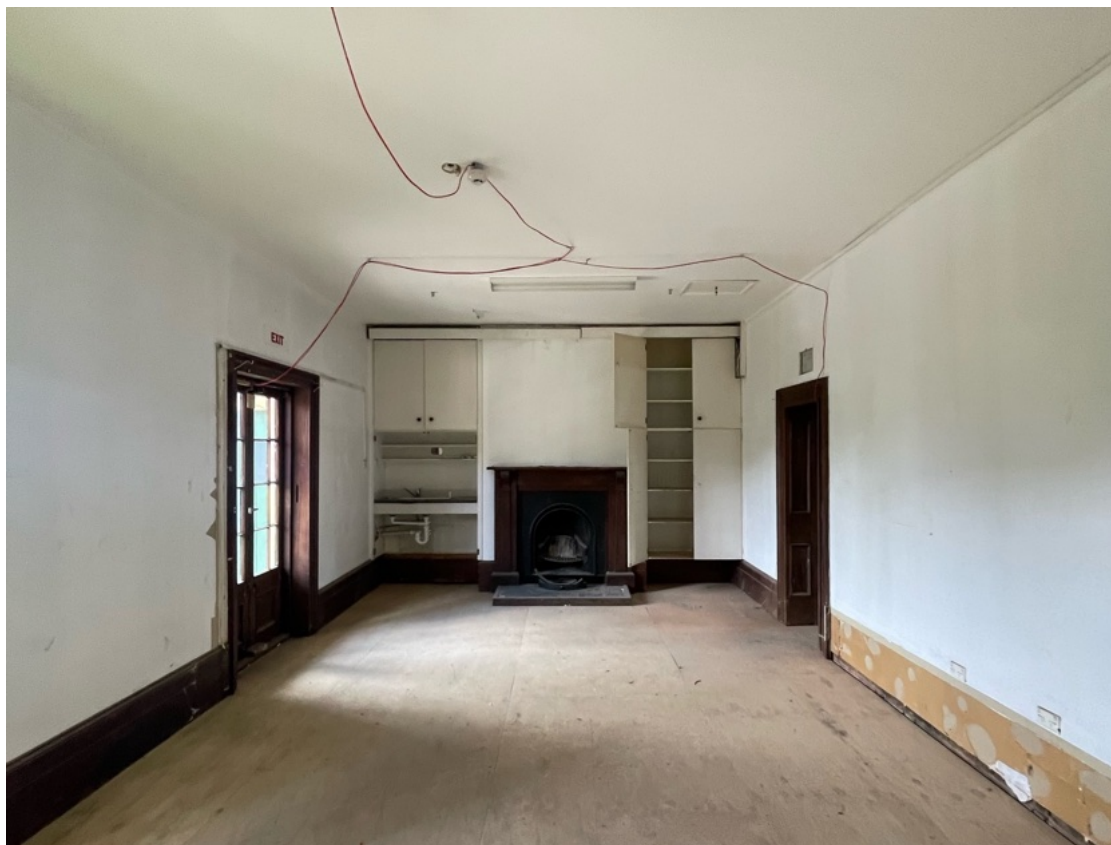
Ground floor rooms have plasterboard walls and ceilings, with no remaining original ceilings above
