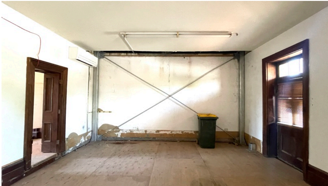
Ground floor rooms after earthquake bracing
