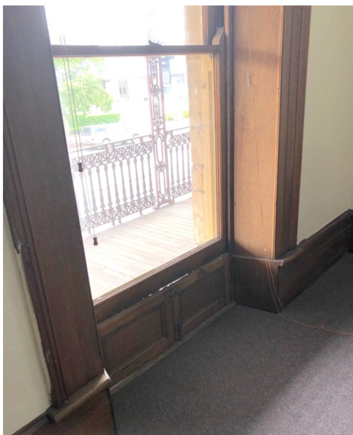
Details of the unusual French 'barn doors' of skirting height that enable an occupant to walk out onto the verandah when the lower sash is raised (L) Patched cedar skirtings below other windows without this original detail (R).
