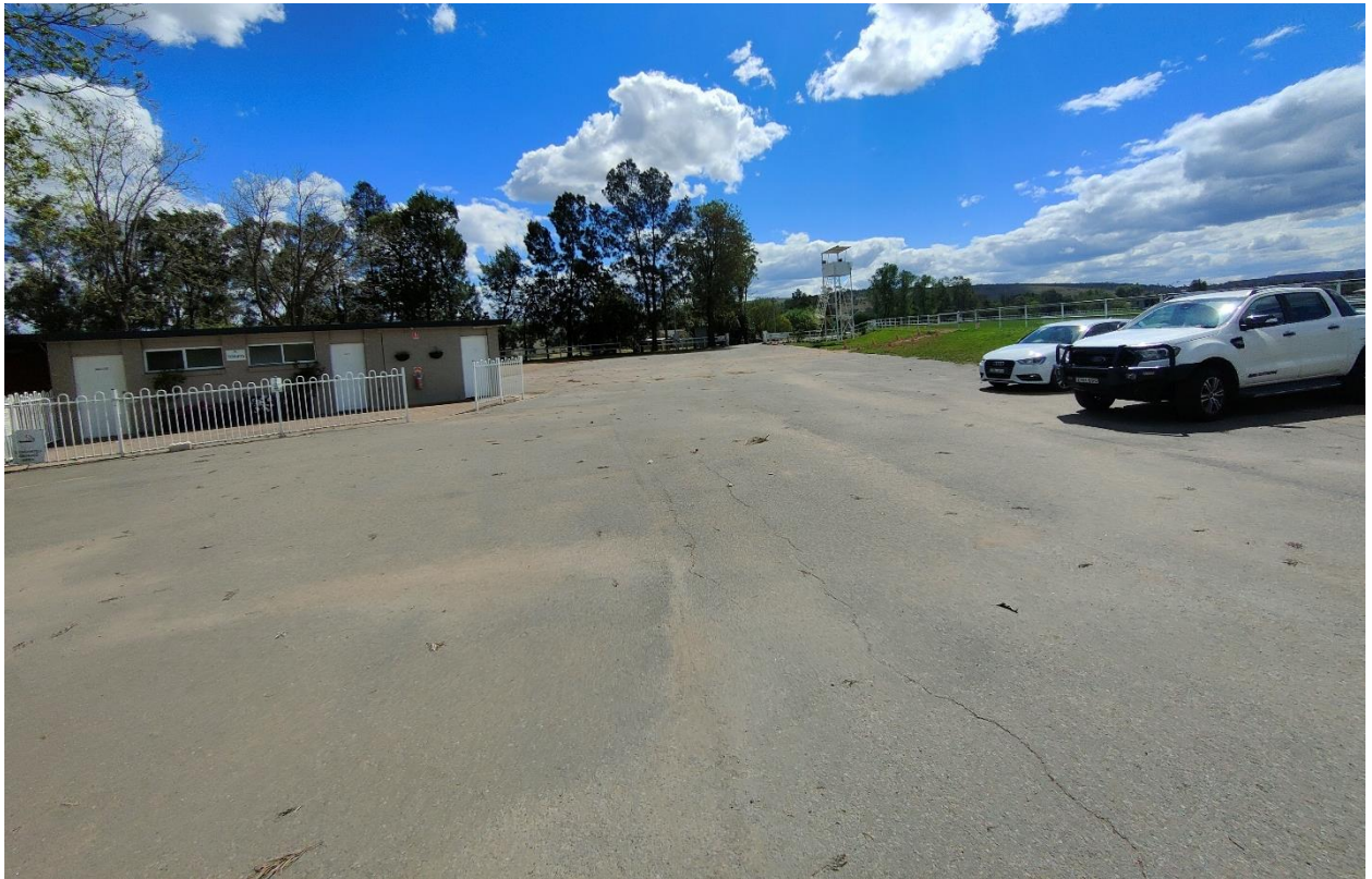
Figure 5 Existing car parking area to the west of the function centre
