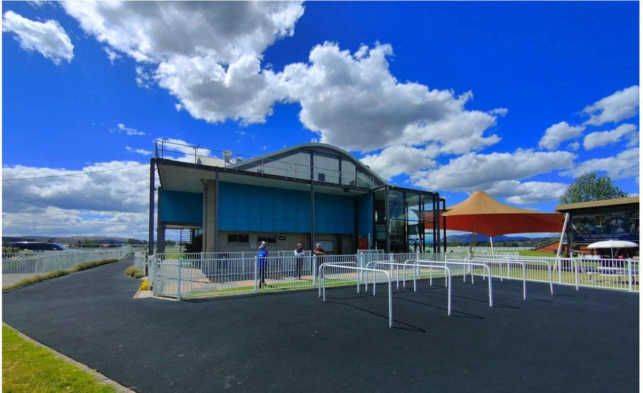
Figure 2 Southern elevation of the existing function centre.
