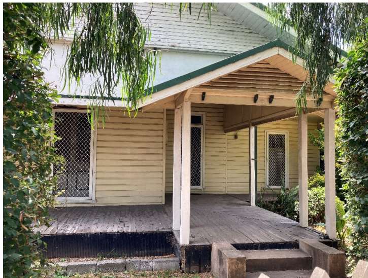
Figure 2 - View of 38 Maitland Street, Muswellbrook, as inspected on the 24/1/2023.
