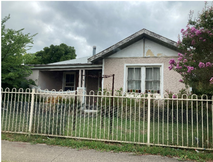
Figure 1 - View of 36 Maitland Road, Muswellbrook, as inspected on the 24/1/2023.
