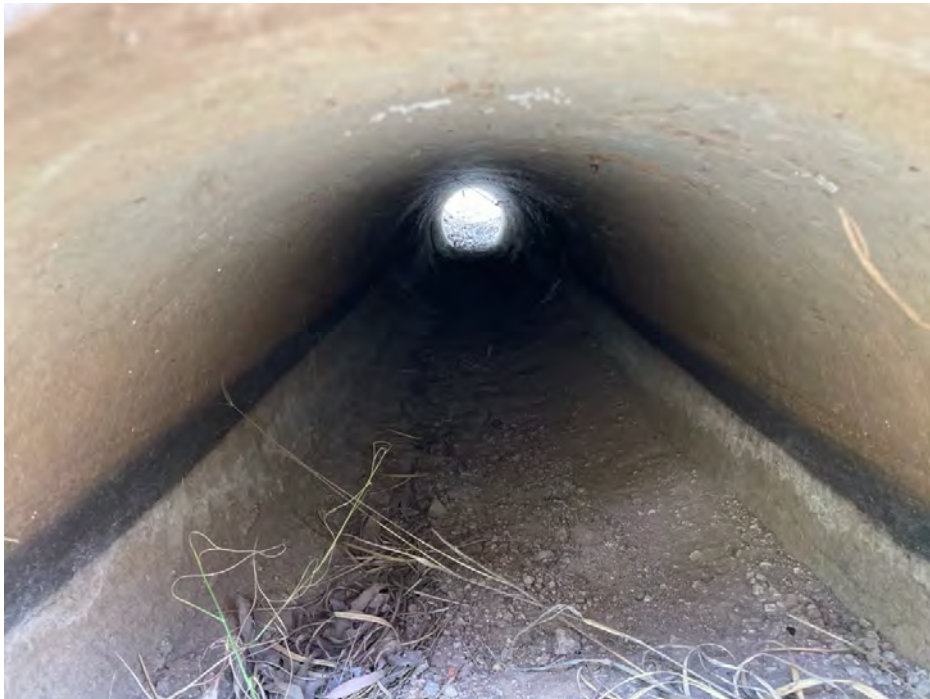
Photo 2: Existing internal condition of a culvert on Bell Street
