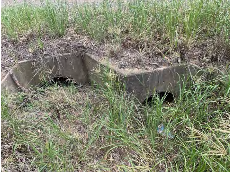
Photo 1: Existing culverts to be cleared and extended
