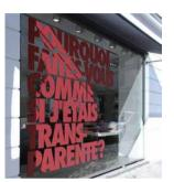
Profile cut coloured SAV applied to the face of the panels with a 2 pack protective clear coat matte finish. Colour to match M4 finish.
