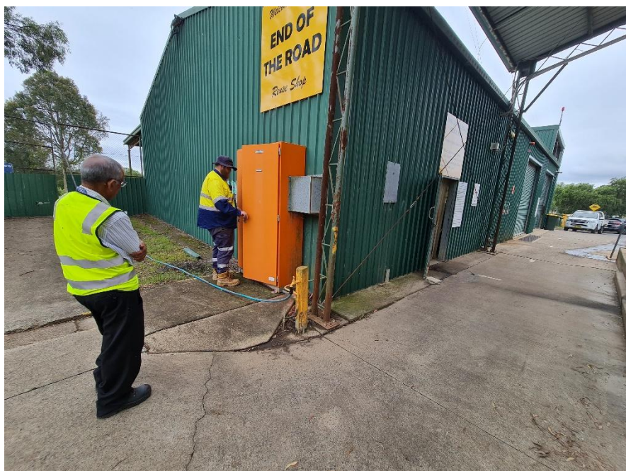
Figure 2, Existing Electrical MSB
