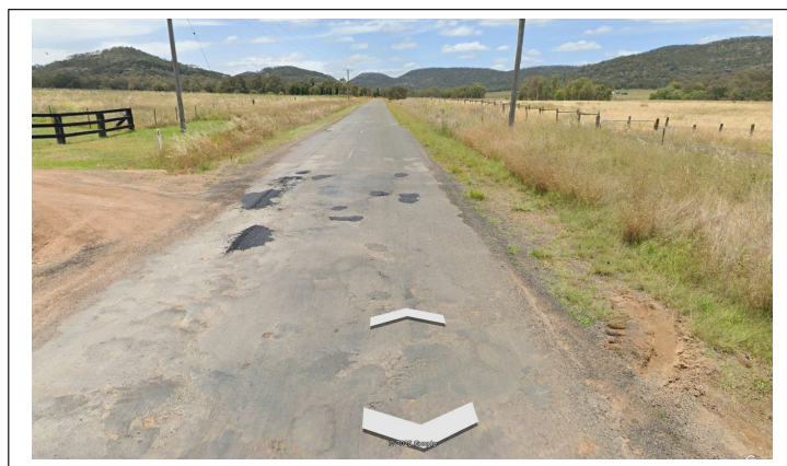
Photo 1 – Google Earth image showing patches, rutting, cracking and flushing near WB9
